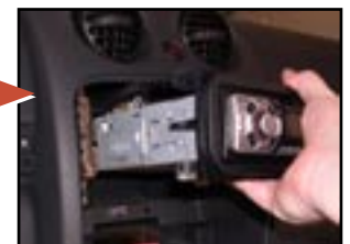
Then the headunit is installed in the kit and the kit gets installed in the dash opening
